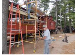
The business car and caboose are getting new roofs! After many months of having a flopping roof and a tarp covered car, the roof and bits of the siding is currently being rebuilt. Sections of siding on the business car are being redone due
